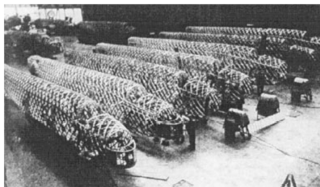
Fig. 3a Vickers geodetic fuselage production.
